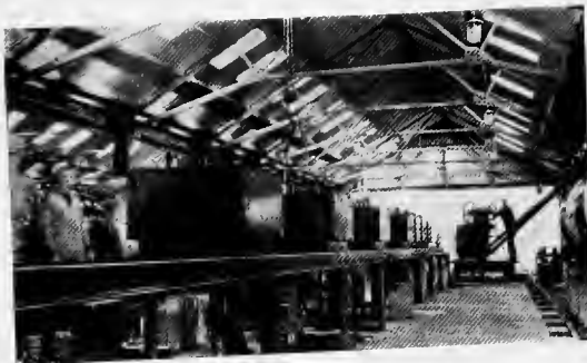
Test Rails for Anchors
